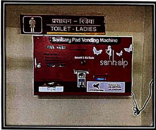
Installed at Ladies Toilet 2 nd Floor
