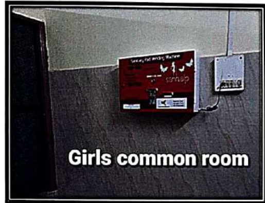
Installed at Girls Common Room
