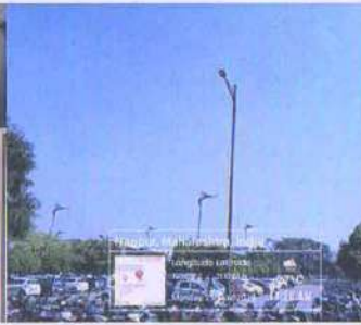
LED lights in Parking
